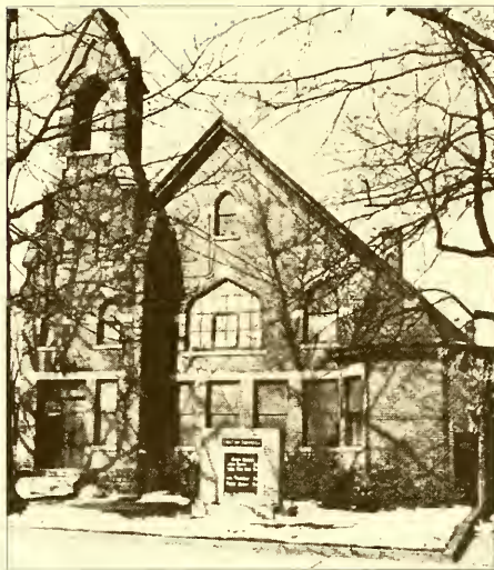
Forest Avenue Baptist Church, shown in undated photograph, before 1940. This building served the Forest Avenue congregation from 1907 until its move in 1940 to the corner of Aycock Street and Walker Avenue. ( College Park Baptist Church )
